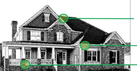
Sloped roof with "broken" roof lines: See 3(b) and 3(c)
